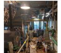
Demolition for boilers and associated work is underway. Electrical rough-ins in progress. Electrical shutdowns began this week, but critical services will have temporary power. Mechanical room asbestos abatement is complete, and selective demolition is ongoing.
