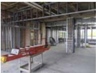
Above ceiling MEP rough-in is ongoing. Wall layout and framing and CMU wall construction is ongoing. Duct work has begun. Project was started two weeks ahead of schedule.
