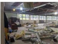
Demolition near completion. Trench layout and excavation has begun. Wall layout has begun. Project commenced approximately three weeks ahead of schedule.
