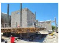
At the addition, bearing CMU masonry walls are in progress. Underground utilities are being installed in preparation for slab on grade pour. In the renovated area, mechanical, electrical and plumbing overhead rough-in and door frames are ongoing. Painting is ongoing. Roofing is in progress; new choral room has been waterproofed.
