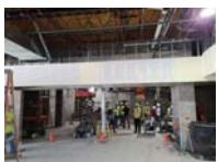
Interior CMU masonry walls are complete. Soffit framing is complete. Drywall, tape, mud, and sand is complete in the cafeteria. Overhead mechanical, electrical and plumbing rough-in is ongoing. Kitchen hoods have been installed; final hookup is underway.
