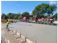
Grandstand structural slab pour and electrical grounding is complete. Ticket booth masonry walls and brick are 25% complete. Ground stabilization is ongoing at the staff parking lot; geogrid will be installed. Mechanical, electrical and plumbing overhead and in-wall rough-in in the classrooms is near completion; painting has begun. Site work for baseball and softball field improvements is underway. Roof replacements are in progress and anticipated to take several weeks; demolition is complete.
