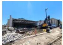
Roof and north exterior wall demolition is complete. Interior demolition is complete. Building foundation, pool shell, and pool deck demolition has begun and is 25% complete. Temporary structure and utility line shoring is ongoing.
